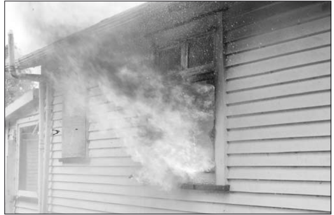
At the point of flashover all the material in a room ignites.
