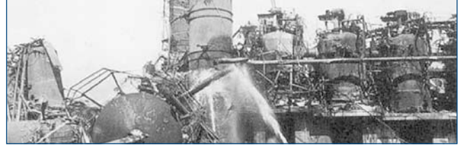
Flixborough (UK) 1 June 1974, 28 workers killed at a chemical plant. The first HAZOP textbook would be written by a member of the accident investigation team and published in 1977.
